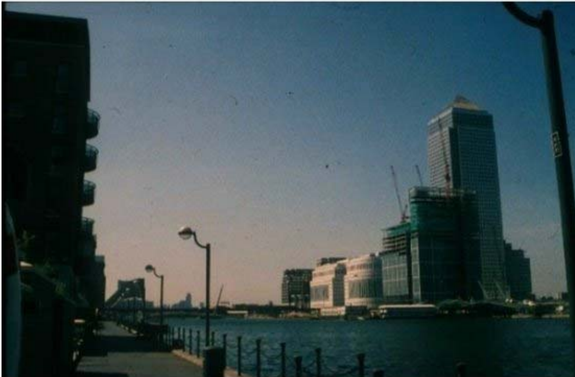
Figure 1: Urban revival: Canary Wharf in Docklands, London, United Kingdom, under construction
