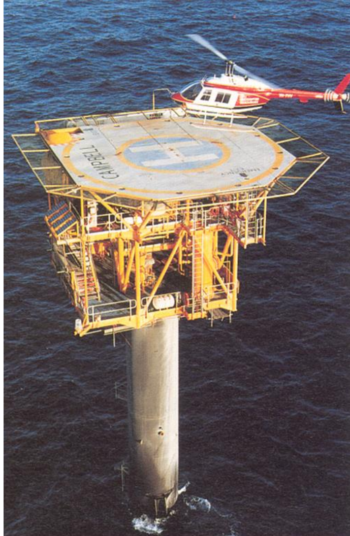
Figure 6. Monotower - here with only one deck with helipad on top
