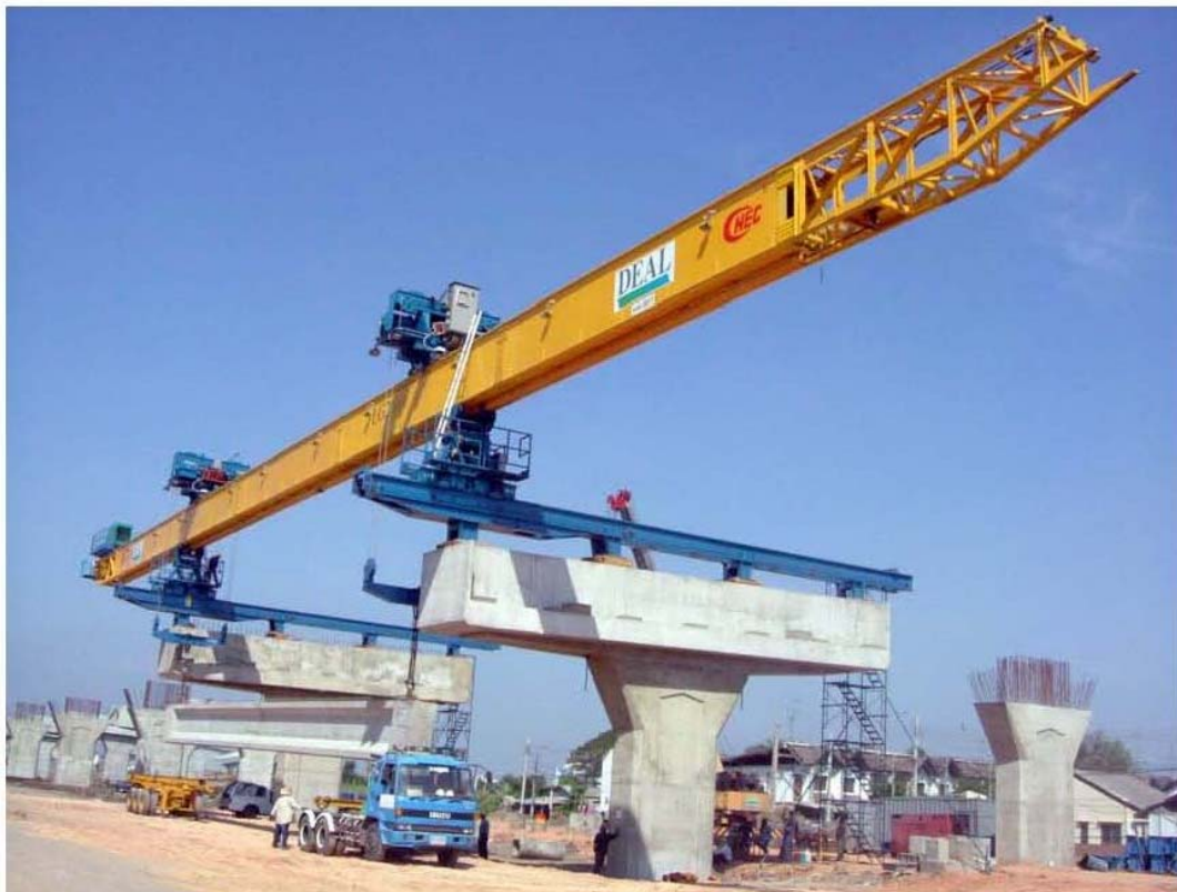
Figure 2. 74m, 98ton single-girder shifter for 28m, 60ton beams (Deal)
