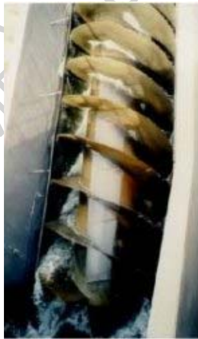
Figure 4: Spiralift™ screw pump. Courtesy of USFilter's Zimpro Products, Rothschild, WI, USA
