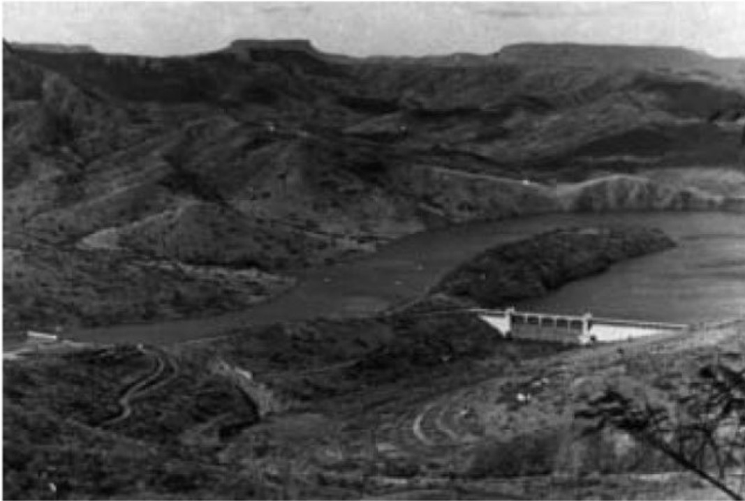
Figure 1. Nagle Dam, Valley of a Thousand Hills, Natal, South Africa (a concrete gravity dam). Note the second dam on the far left. This controls the flow into the reservoir and acts as a silt trap. Excess flow and silt can be removed through a sluice to the right of this dam, the water and silt flowing through a cutting into the river below Nagle Dam.
