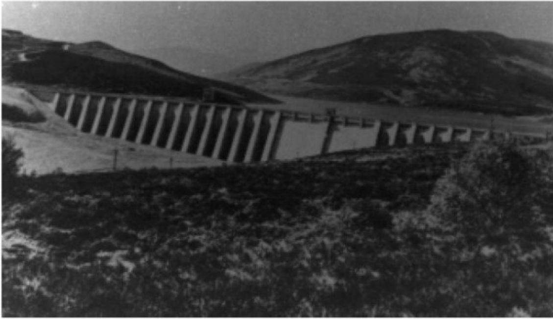
Figure 3. Errochty Dam, Scotland (a buttress dam)
