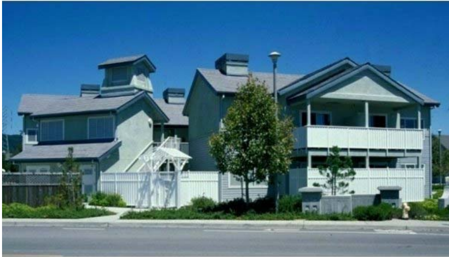
Figure 1: Ecology House, San Rafael, California. Kodama Associates, Architects. Photograph by the author.
