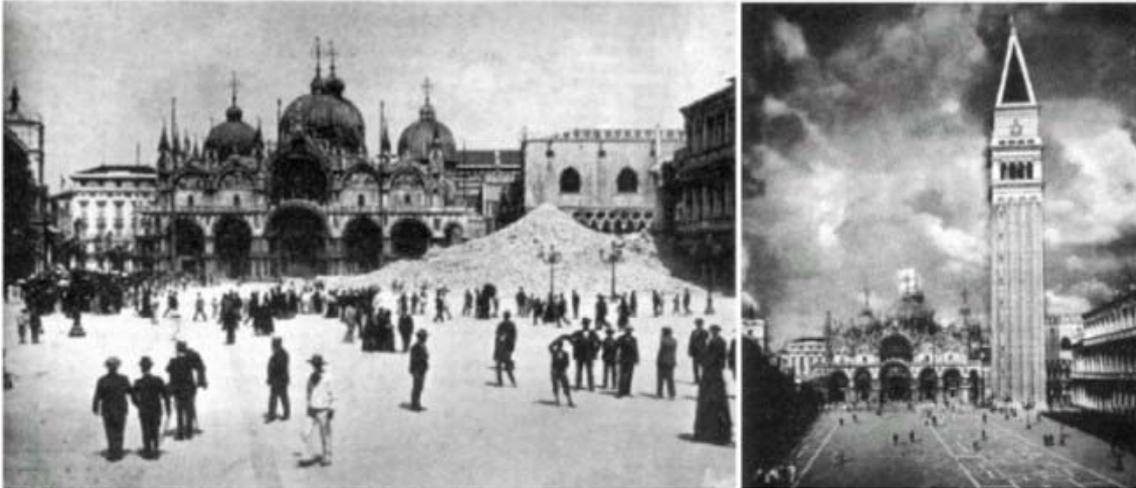
Fig. 1-2 Venice (Italy) the spire of San Marco, the first instance of reconstruction “as it was, where it was”. The remains of the old spire, that collapsed on 14 July 1902 (left) and the new spire (1912) identical to the earlier one, but only externally, the interior structure having been reconstructed with r.c.
