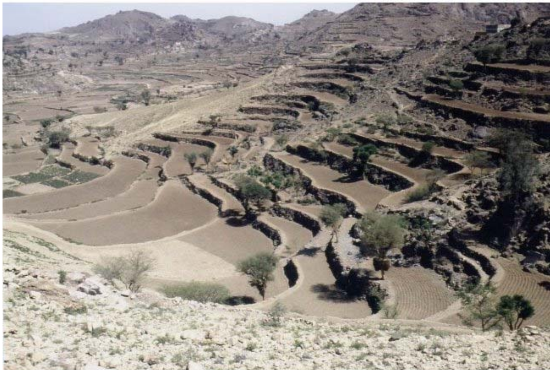
Figure 2. Beautifully built terraces in Yemen carefully maintained over the centuries
