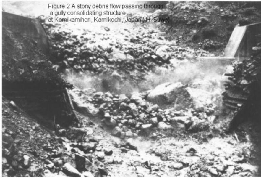
Figure 2. A stony debris flow passing through a gully consolidating structure at Kamikamihori, Kamikochi, Japan
