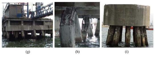
Figure 2. Observed pile damages in recent earthquakes
