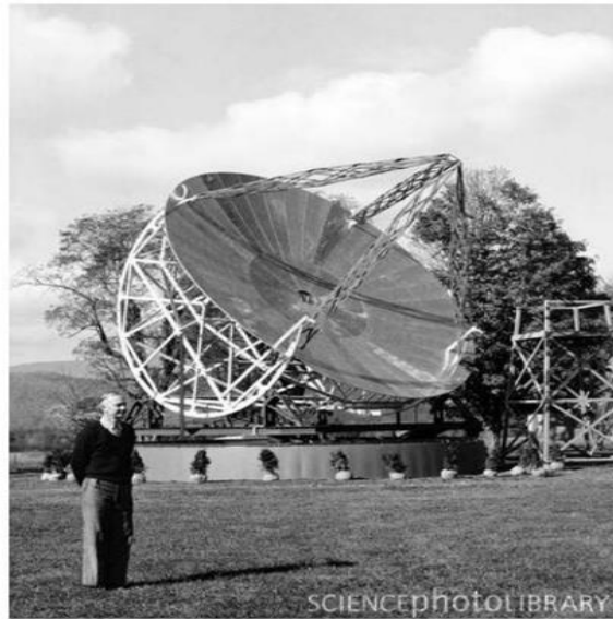
Figure 4. Reber radiotelescope in Wheaton, Illinois, in 1937. (Credit: Emilio Segre Visual Archives/American Institute of Physics/Science Photo Library).
