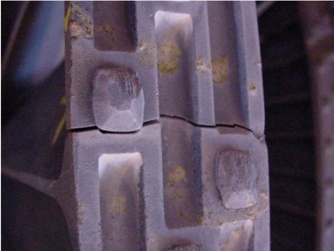
Figure 1. A crack in the shroud of a low pressure steam turbine. Reproduced by permission of Innogy plc.
