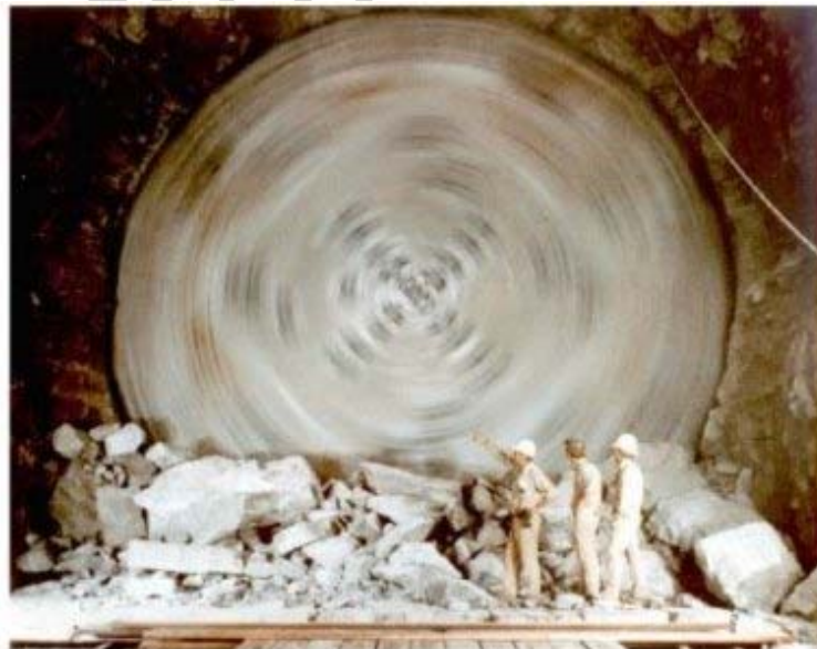
Figure 2: Chicago Tunnel and Reservoir Plan (TARP) 9.76-m diameter Tunnel Boring Machine. Courtesy of Harza Engineering Co., Chicago, IL.
