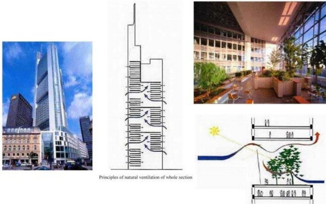
Figure 3. The tallest building in Europe using natural ventilation. General view of the building (left), building cross section and outline of natural ventilation and stack effects (center), detail of the court yards viewed from inside (top right picture), and cross section and outline of natural ventilation (bottom right picture) [Source: Commerzbank, 2000.]
