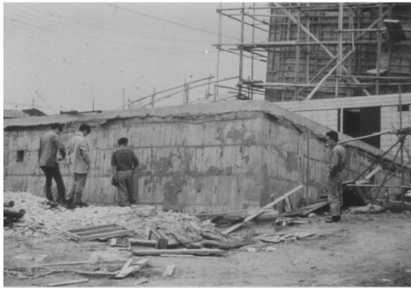
Figure 2. Uplift of Underground Structure
