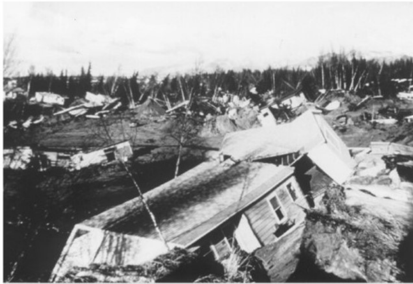
Figure 5. Landslide at Ternagen Hight (after H. B. Seed)
