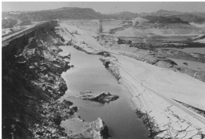
Figure 4. Upstream Slide of the Lower San Fernando Dam (after H. B. Seed)
