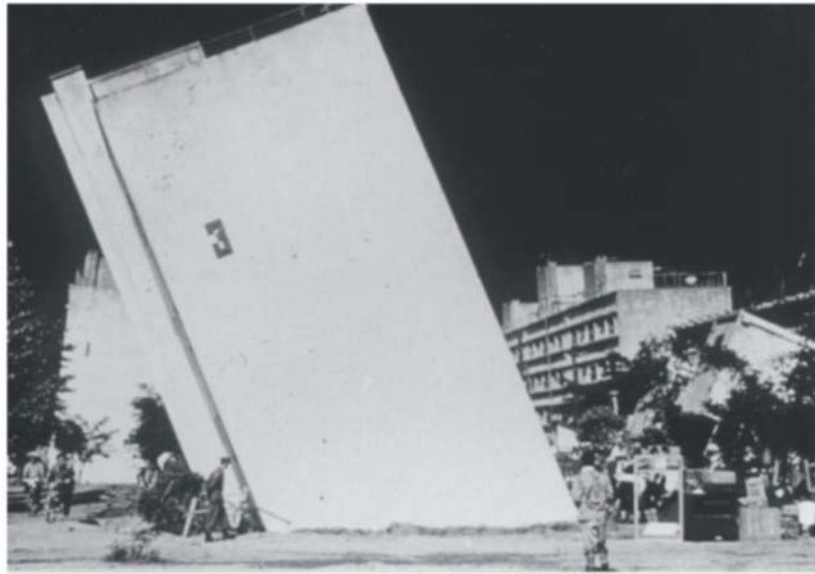
Figure 1. Liquefaction-induced Bearing Failures
