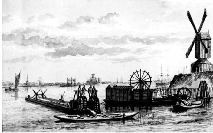
Figure 6. Mud-mills in operation. One is driven by a human treadmill, a second driven by horsepower
