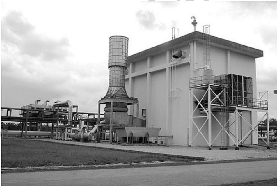
Figure 1 – An Example of a Compressor Station
