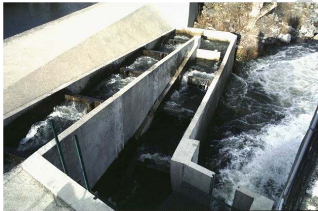
Figure 1. An example of a fish pass (successive pools), EDF hydro-electric power plant (Loire River, Brives-Charensac, France). (Photo: H. Carmié – Photothèque CSP).
