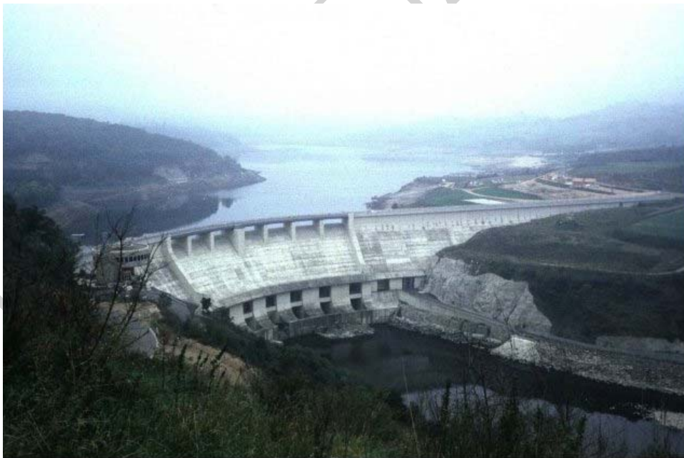
Figure 4. Villerest Dam on the River Loire. In addition to the impediment to fish movement note the impact on the river morphodynamics upstream and downstream of the dam.
