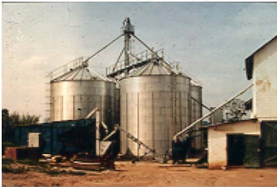
Figure 3. Corrugated steel silos for grain storage.
