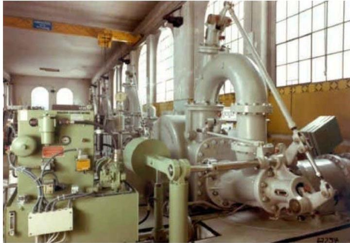
Figure 4. Modernized turbine control system (1986) at Burglauenen (Jungfrauoch-Bahn, Switzerland, four two jet Pelton units 1 MW each), left hand foreground: pressure oil subsystem, center: servomotor supporting the closing weight, actuating the two needles by the lever arrangement, right background: closing weight for the shutdown valve
