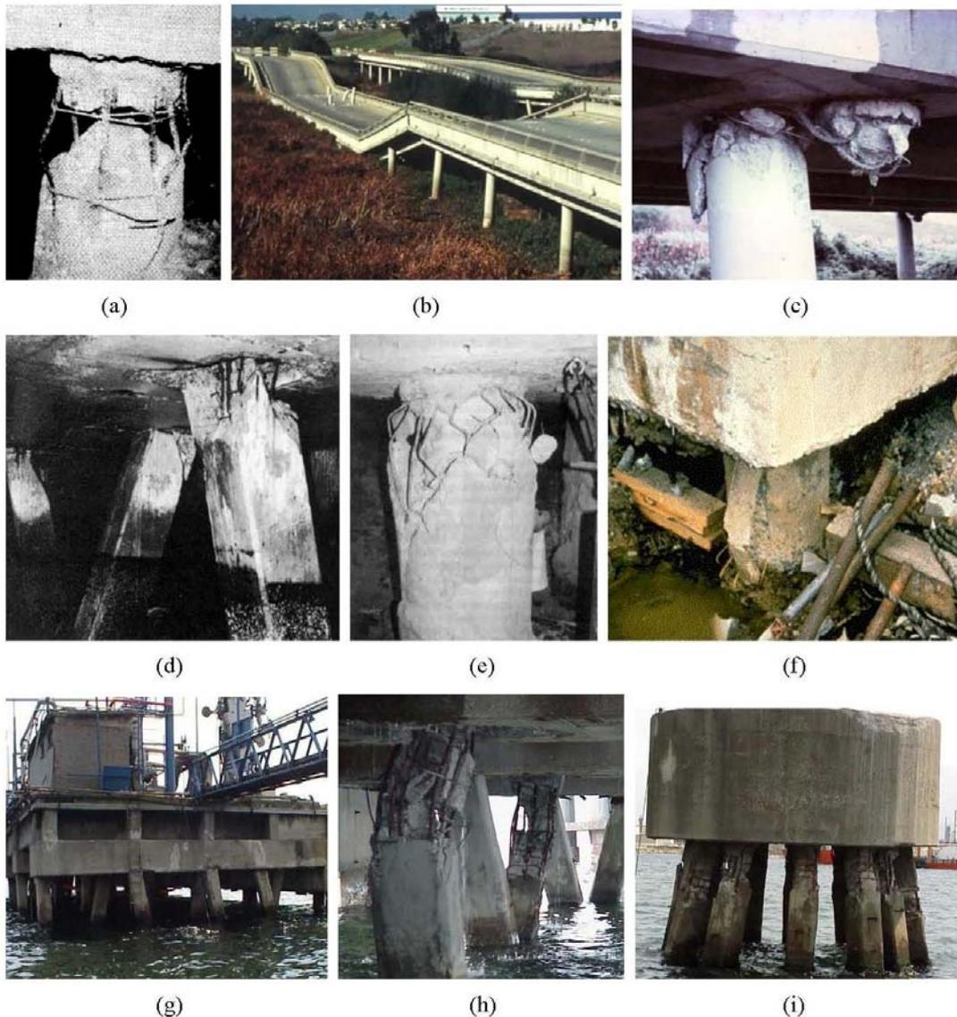
Figure 2. Observed pile damages in recent earthquakes
