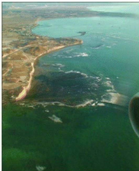
Plate 1. Cliffs and abrasion platforms characterize the Patagonian coast. Caleta Córdova is a village oriented to petroleum production close to Comodoro Rivadavia city, Chubut. Coastal facilities, such as jetties and pipelines, affect coastal dynamics and cause more erosion.
