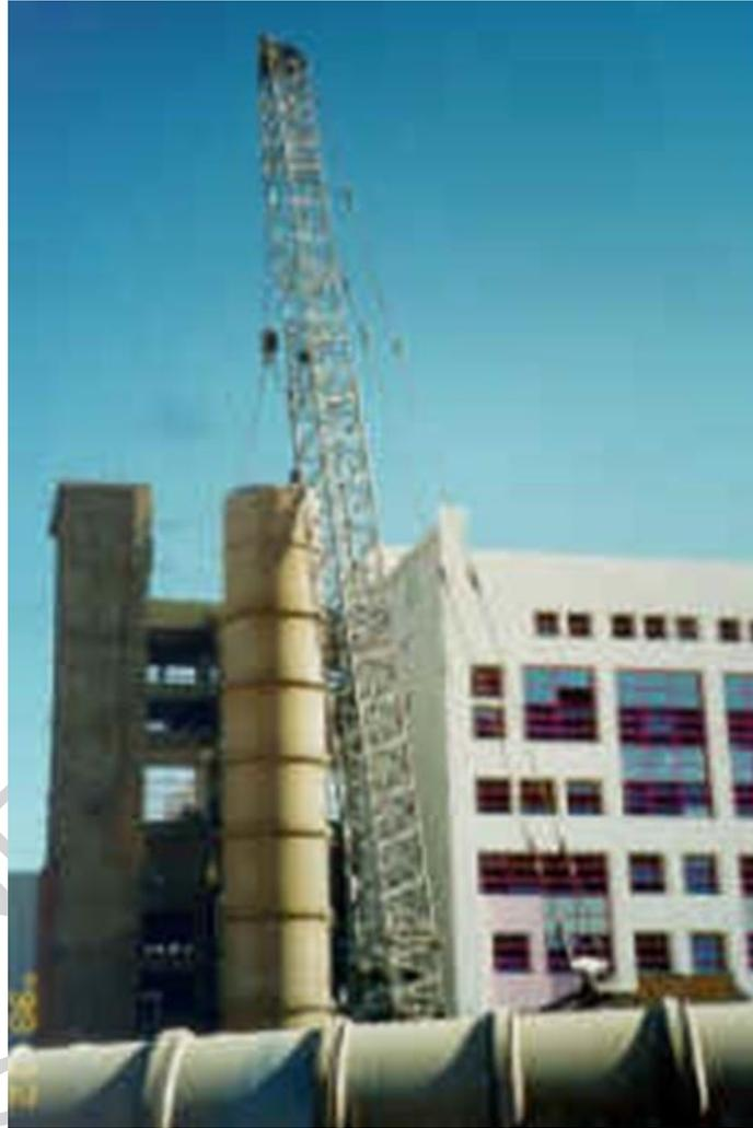
Figure 3. Citric acid production reactors during their erection (Photo Courtesy of Vogelbusch Vienna)
