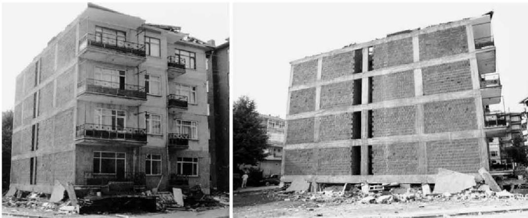
Figure 7. First two stories collapsed building – Kocaeli earthquake (photos by K. Mosalam)
