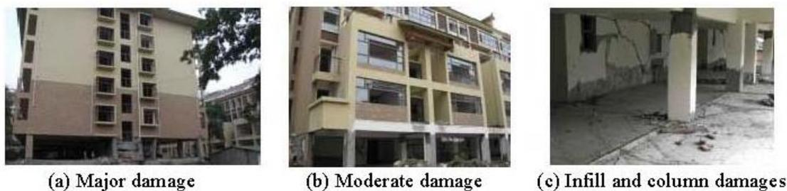
Figure 2. Effect of the lack of first story infill walls on damage – Wenchuan earthquake (photos by B. Li)
