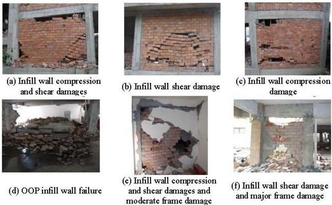
Figure 3. Damage of URM infilled RC frames – Wenchuan earthquake (photos by B. Li)
