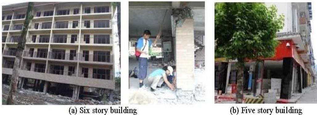
Figure1. First story damaged buildings – Wenchuan earthquake (photos by K. Mosalam)
