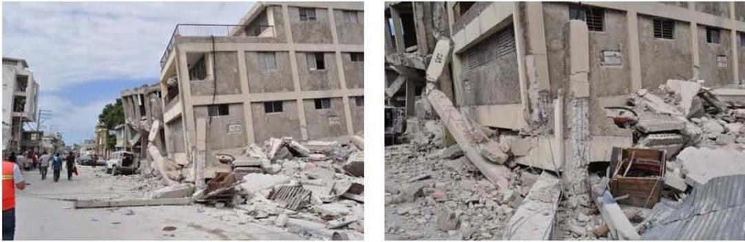
Figure 8. First story collapsed building – Haiti earthquake (photos by E. Fierro)
