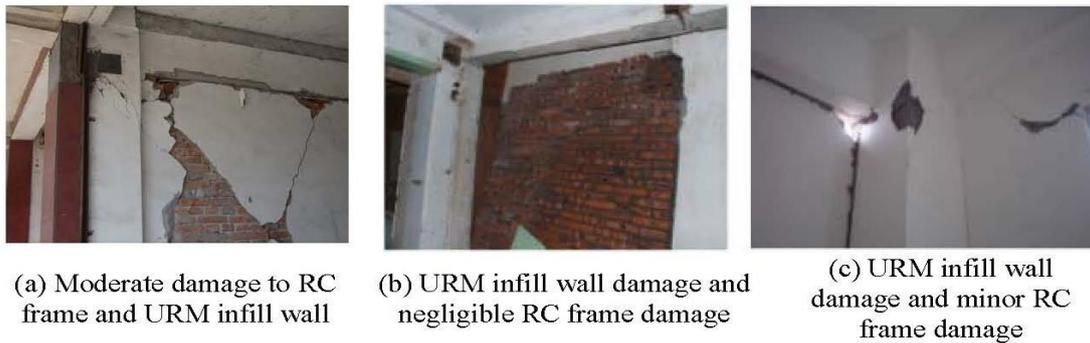
Figure 4. Frame-infill wall interaction – Wenchuan earthquake (photos by B. Li)
