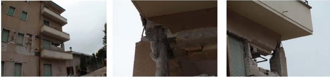
Figure 6. Joint failure due to infill damage – L'Aquila earthquake (photos by K. Mosalam)
