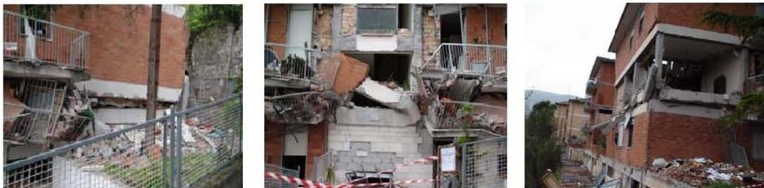
Figure 5. Story collapse due to infill failure – L'Aquila earthquake (photos by K. Mosalam)
