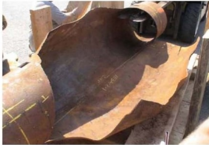
Figure 2. Steam pipe at municipal heating system that ruptured because of severe load imposed by water hammer event.
