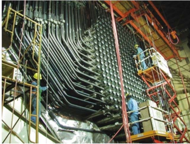
Figure 4. Feeder tube assembly on reactor face
