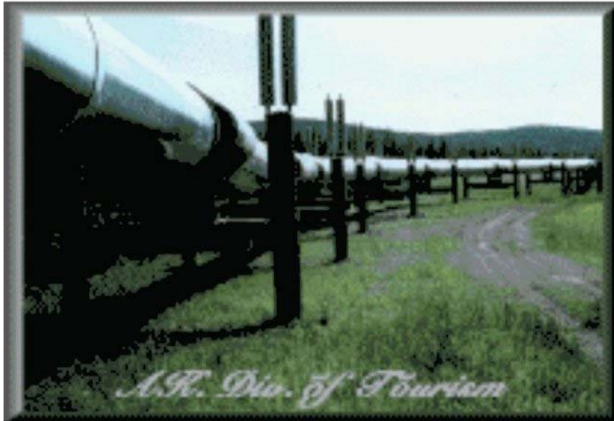
Figure 2. The Trans-Alaska pipeline.
