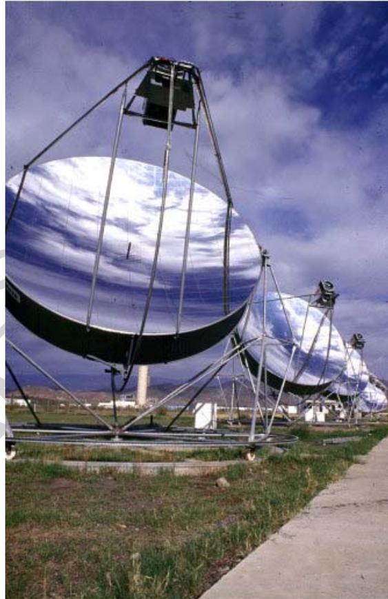
Figure 2. High concentration solar collector. Parabolic dish solar reactor (PSA, Spain)
