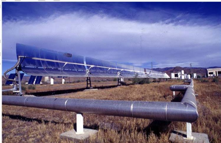
Figure 1. Medium concentration solar collector. One-axis parabolic trough collector (PSA, Spain)
