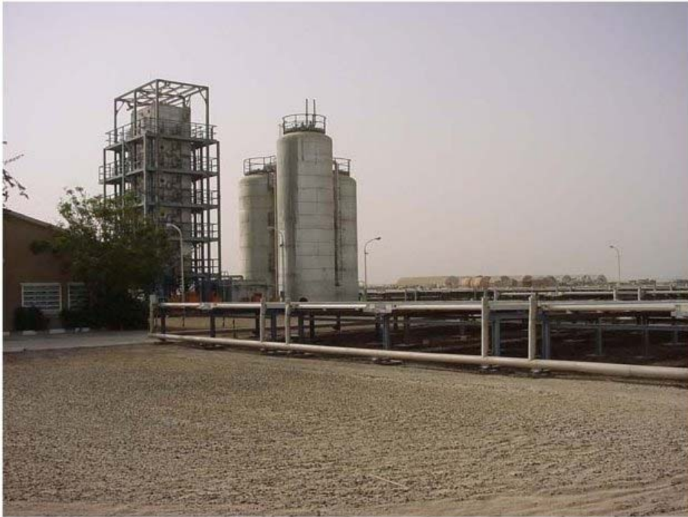
Figure 1 Picture of Abu Dhabi solar desalination plant
