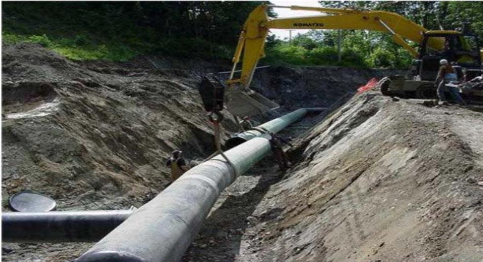
Figure 2. Open cut installation of buried pipelines.
