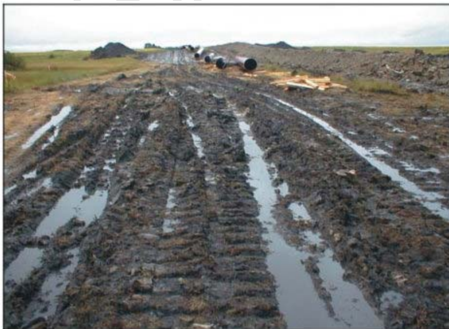
Figure 2. Wet Weather Shutdown of Construction Activities along Right-of-Way
